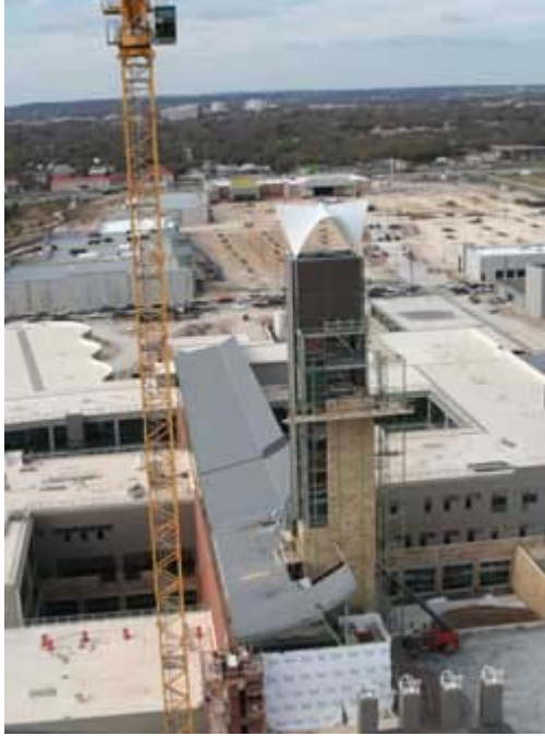
Photo courtesy White Construction Co.
